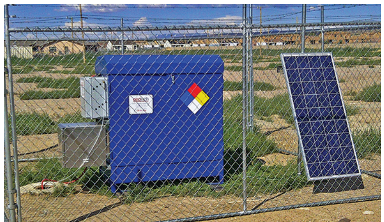
Solar Sipper installation mounted on hazmat enclosure
